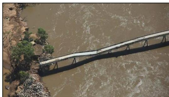
Image 2: Damaged Bridge into Fitzroy Crossing<sup>2</sup>
