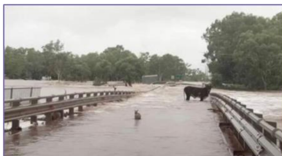
Image 1: Fitzroy Crossing Bridge during flood 1
